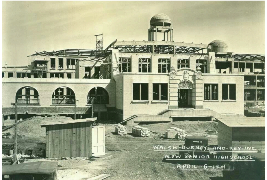
The yet-to-be-named "New High School," under construction in 1931.
