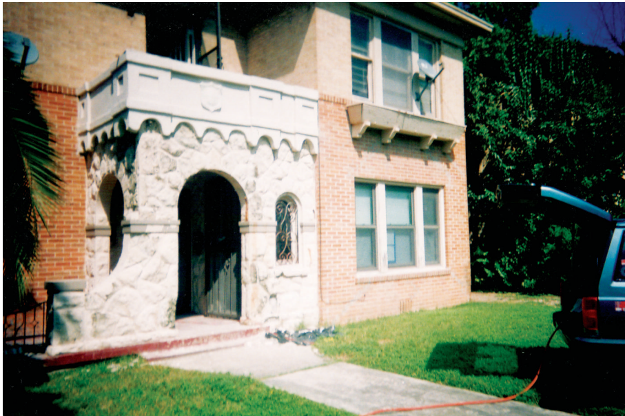
Bob Howard expertly restored the masonry at 507 Furr Drive
