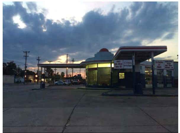
Photo #1, What is at 2202 Fredericksburg Road
