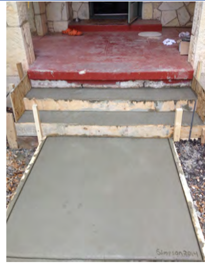
The work in progress
